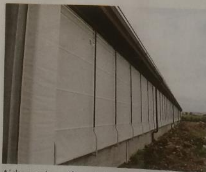
Airkoe automatic curtain system has been fitted to one side of the shed, allowing control of the temperature during winter.
