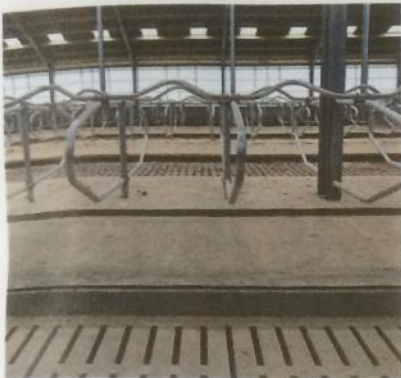
Veitch-designed cubicles and the cranked neck rail are made by IAE. Rather than fitting a brisket board, a stepped concrete central section was used at Myremill.
