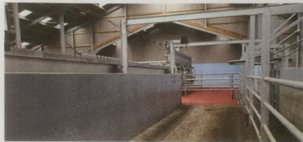
Rubber paint has been applied to all the walls in the handling area to make cleaning easier. More costly Duraflake resin was used in the parlour pit and dairy.
