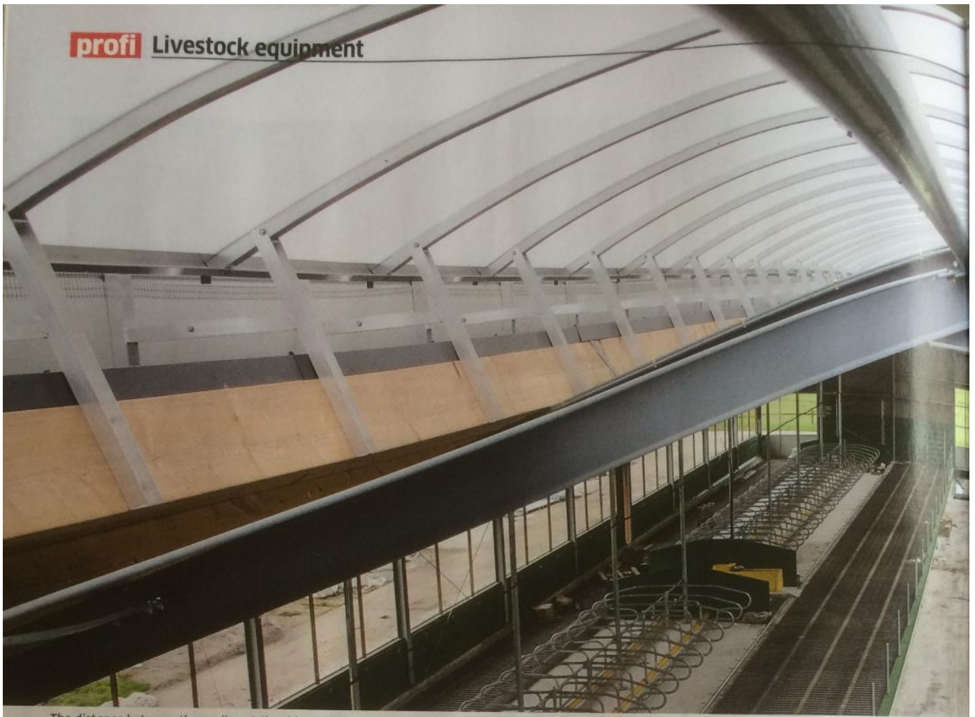
The distance between the purlins at the ridge will determine the width of the ridge. The ridge can be retrofitted, though this is a more expensive route. Ball park figures are £140-190/m depending on the width and span, which can range from 1.5m to 4.0m.
